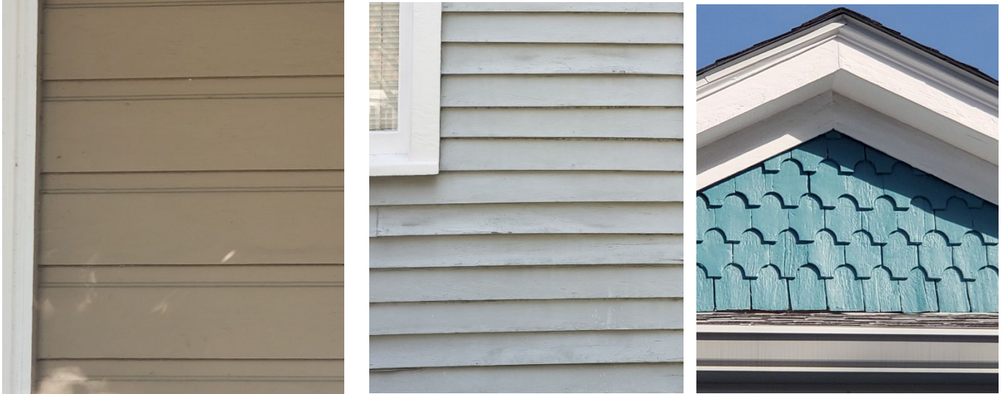
Figure 14: Examples of various types of wooden siding - drop siding (L), clapboards (center), and decorative shingles (R).
