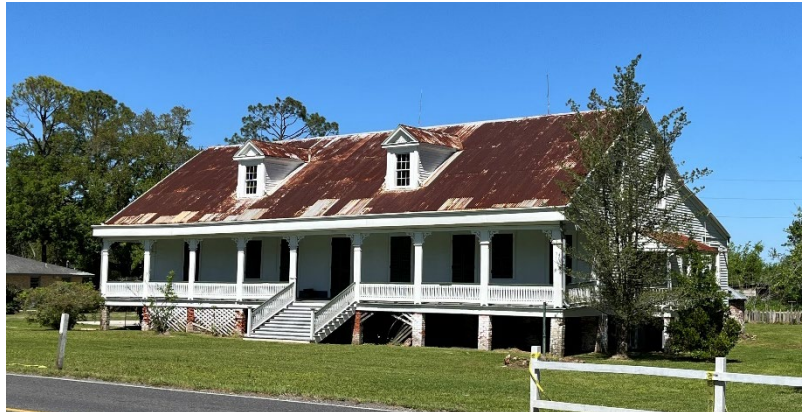
Figure 5: Bonnet Carre Historical Society / Kid Ory House on LA Hwy 628.
