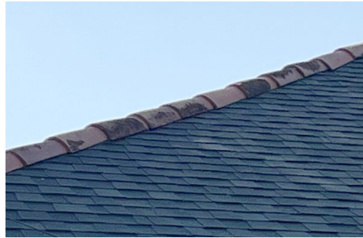
Figure 9: Example of a ridge tiles on an asphalt roof
