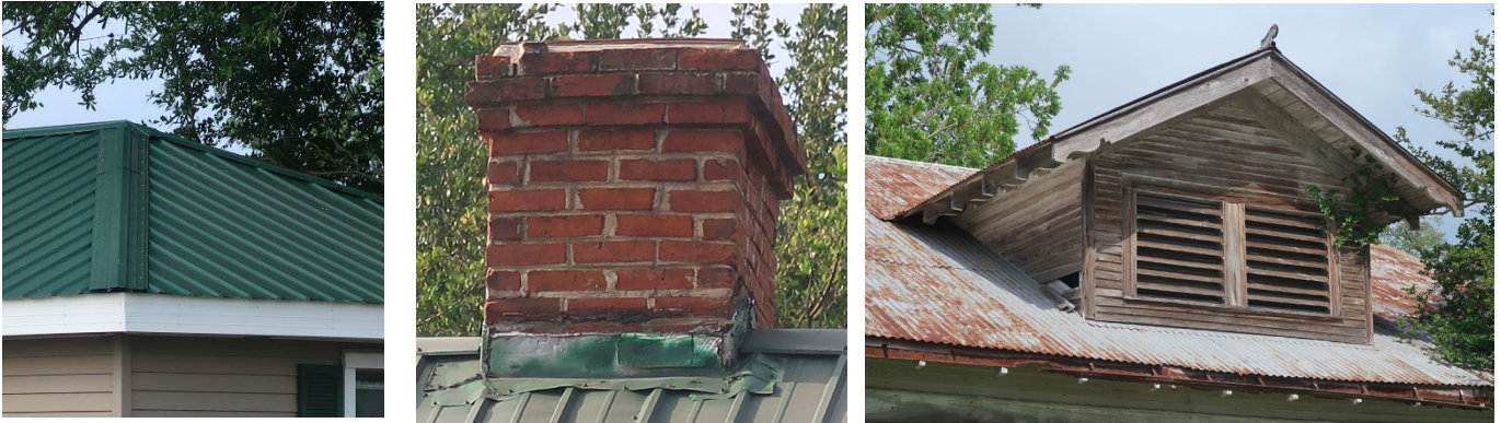
Figure 12: Examples of a modern metal roof, brick chimney, and dormer.
