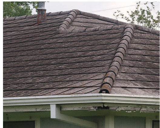
Figure 10: Example of an asbestos shingle roof
