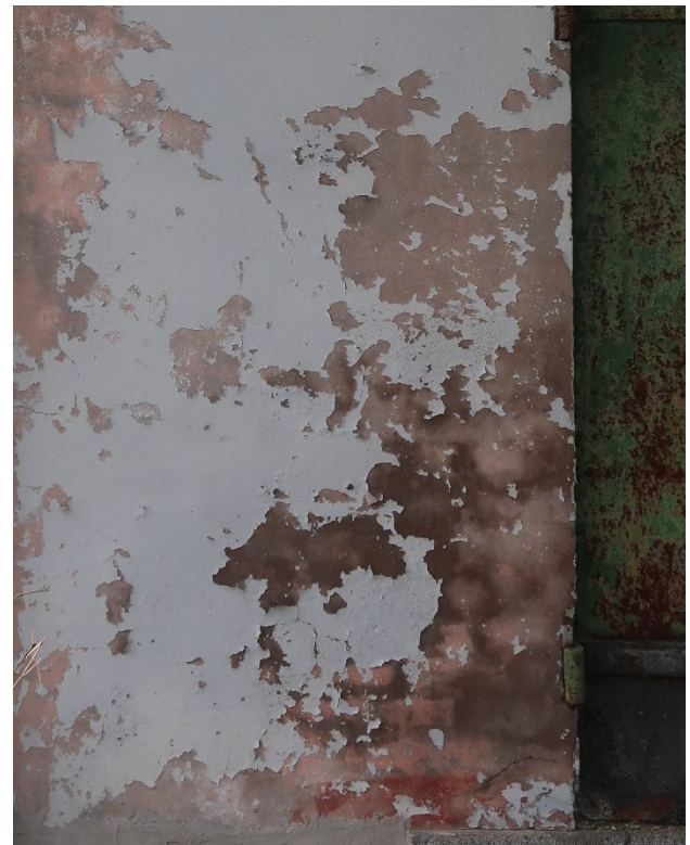
Figure 16: Detail of a stucco clad wall
