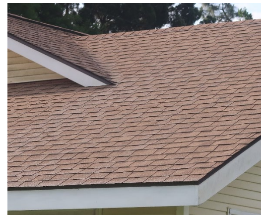
Figure 11: Example of an asphalt shingle roof.
