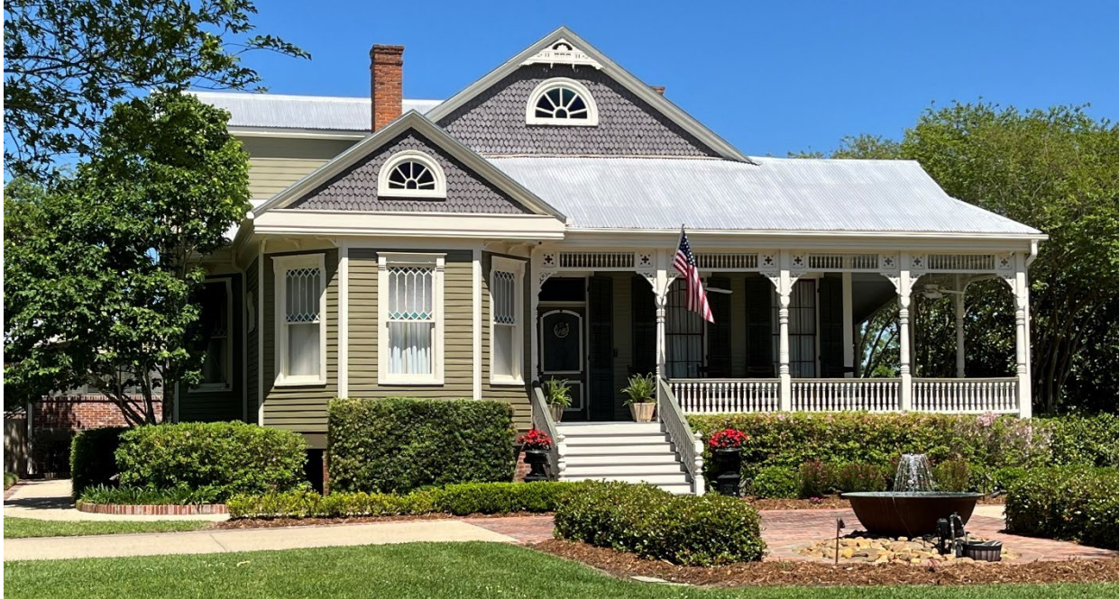
Figure 20: A porch with intact historic details.
