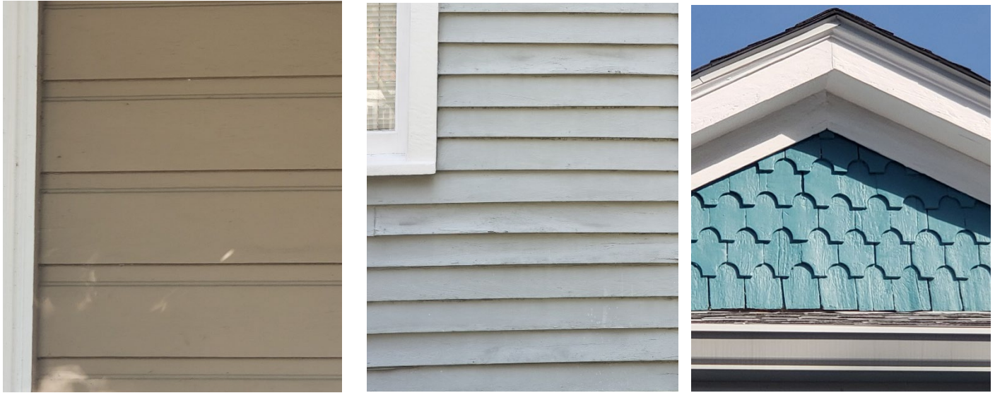
Figure 12: Examples of various types of wooden siding - drop siding (L), clapboards (center), and decorative shingles (R).
