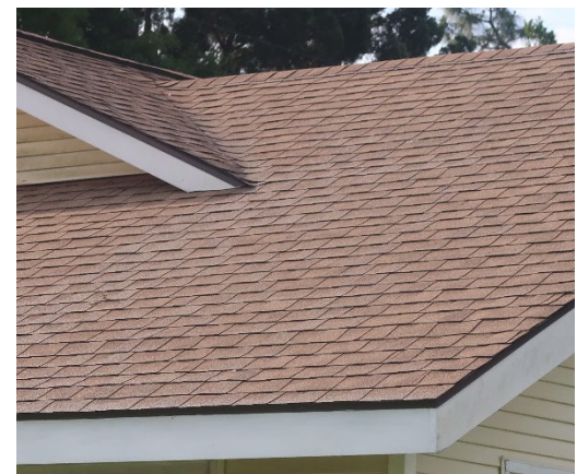
Figure 9: Example of an asphalt shingle roof.
