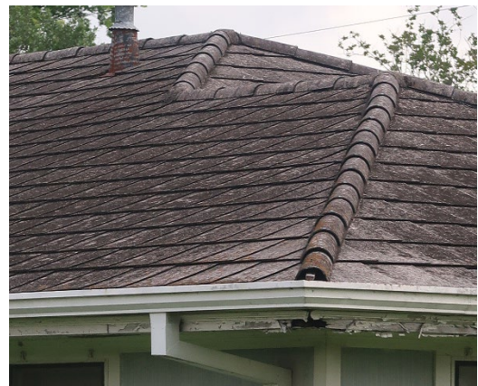
Figure 8: Example of an asbestos shingle roof
