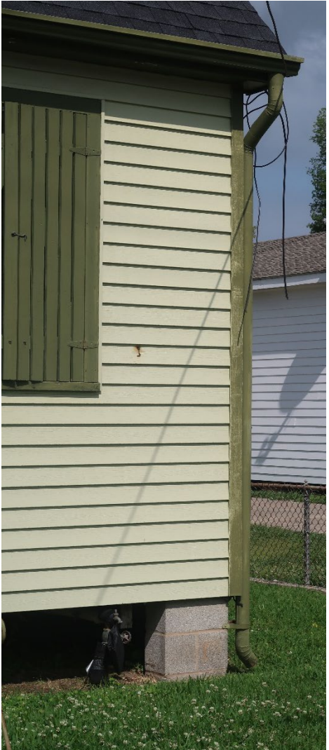
Figure 11: Example of a gutter and downspout
