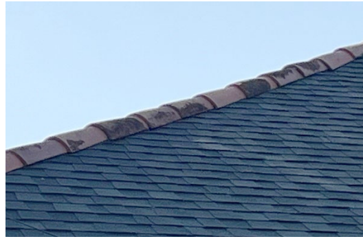
Figure 10: Example of a ridge tiles on an asphalt roof
