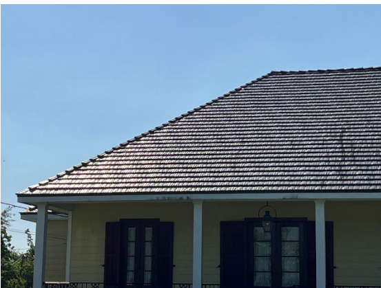
Figure 9: Example of synthetic slate roof
