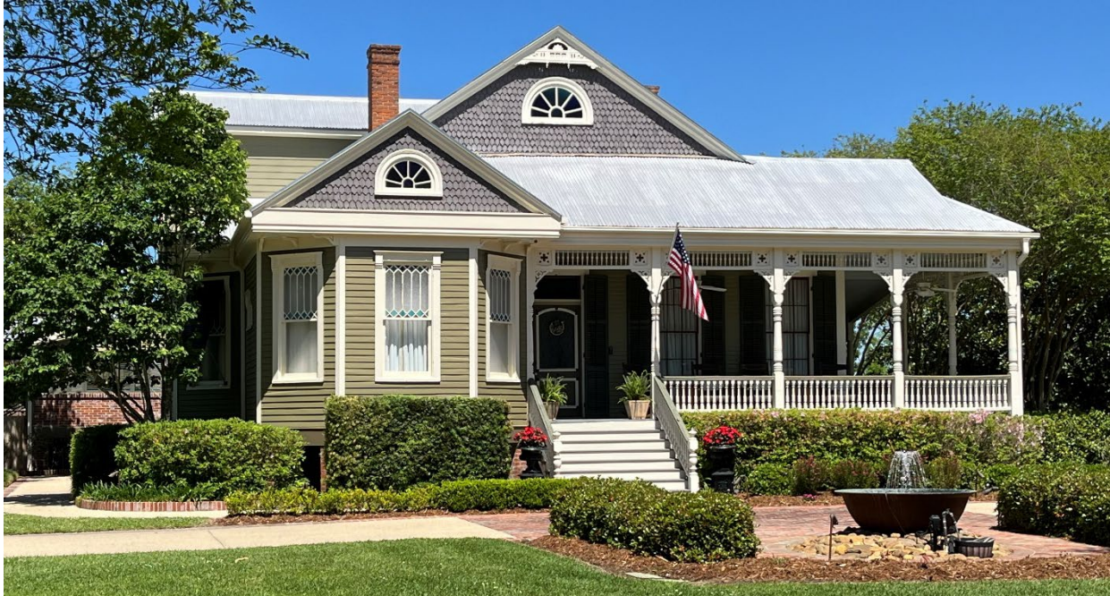
Figure 21: A porch with intact historic details.
