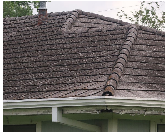
Figure 11: Example of an asbestos shingle roof
