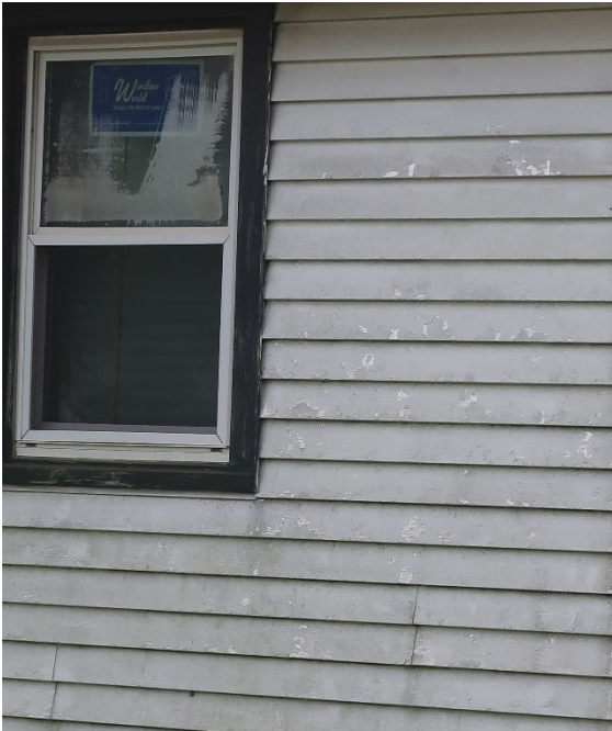
Figure 18: Example of aluminum siding (L) and asbestos shingle siding (R)
