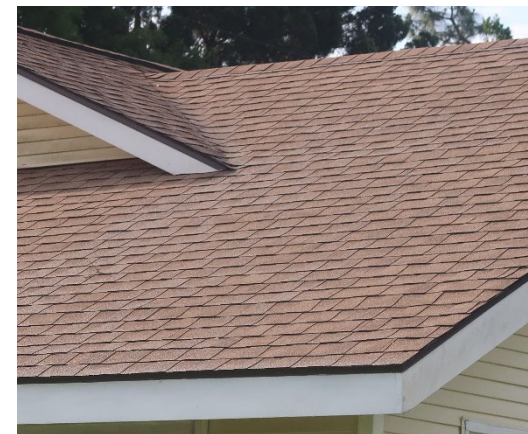
Figure 12: Example of an asphalt shingle roof.
