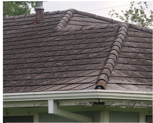
Figure 9: Example of an asbestos shingle roof
