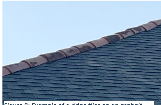
Figure 8: Example of a ridge tiles on an asphalt roof
