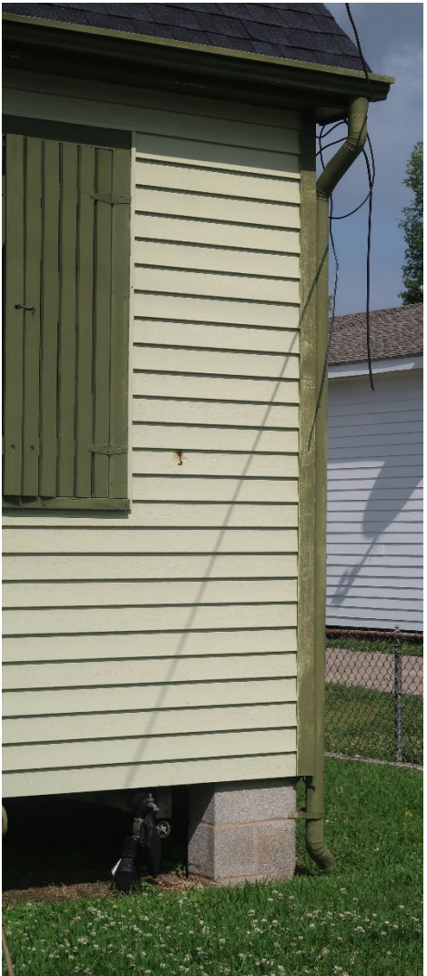
Figure 12: Example of a gutter and downspout
