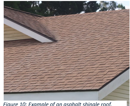
Figure 10: Example of an asphalt shingle roof.
