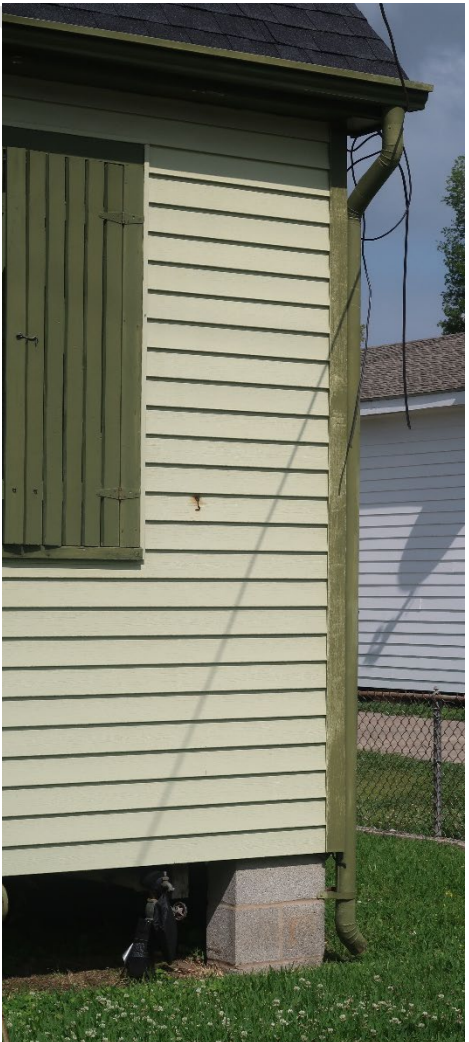
Figure 16: Example of a gutter and downspout
