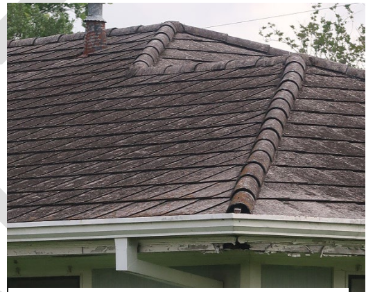
Figure 13: Example of an asbestos shingle roof
