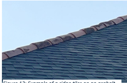
Figure 12: Example of a ridge tiles on an asphalt roof
