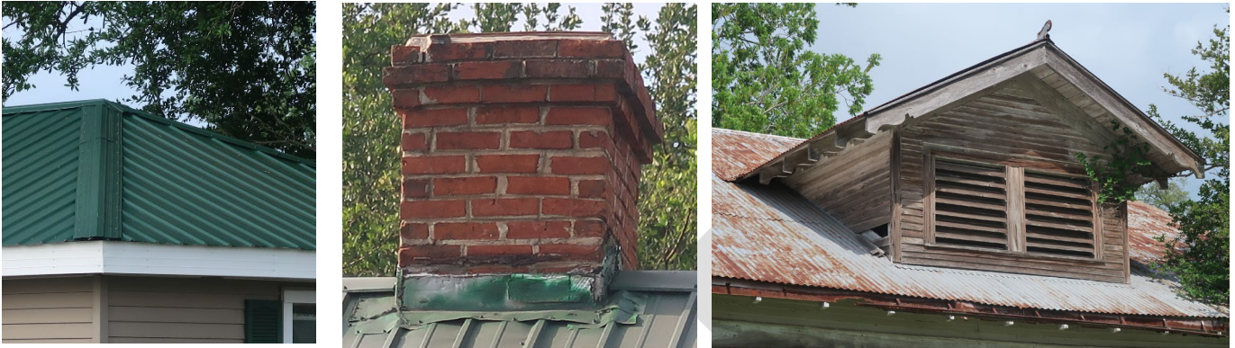
Figure 15: Examples of a modern metal roof, brick chimney, and dormer.
