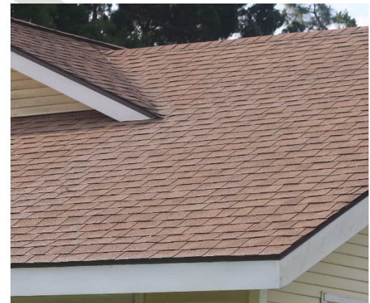
Figure 14: Example of an asphalt shingle roof.
