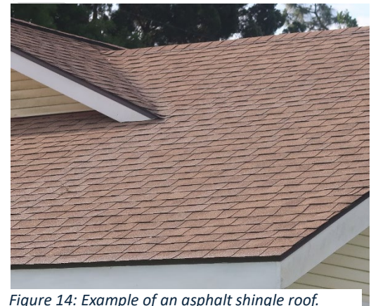
Figure 14: Example of an asphalt shingle roof.
