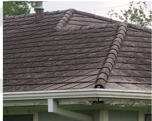
Figure 13: Example of an asbestos shingle roof
