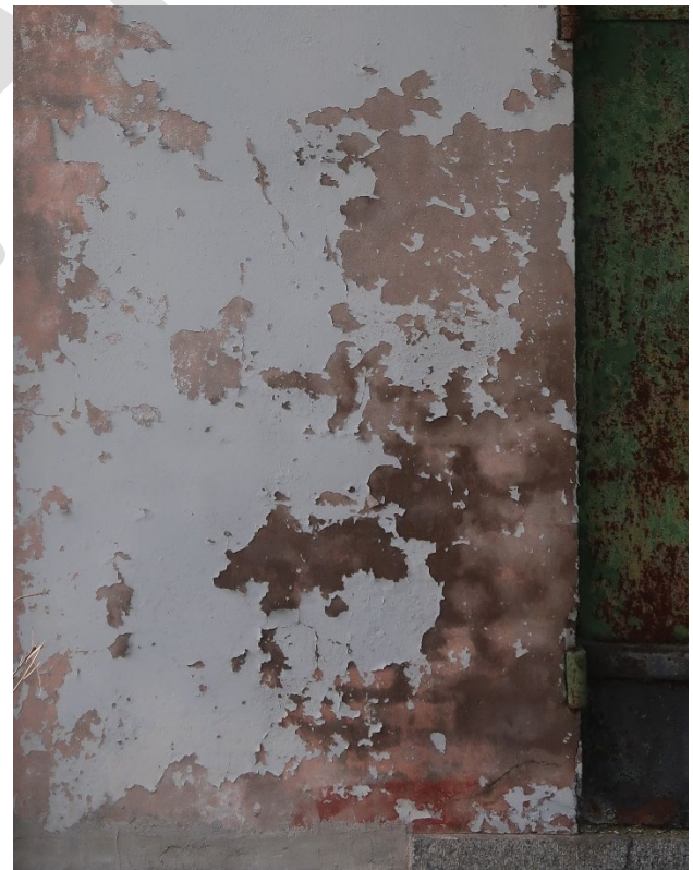
Figure 19: Detail of a stucco clad wall
