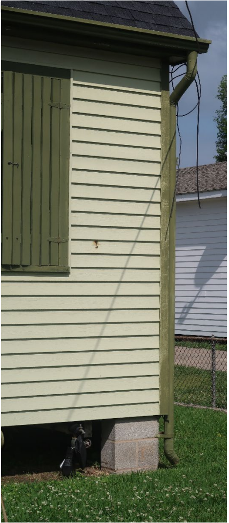
Figure 23: Example of a gutter and downspout
