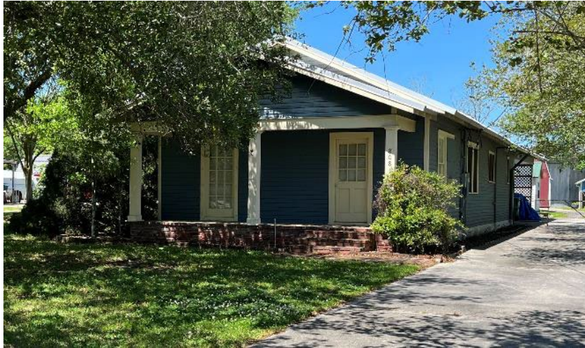
Figure 4- c.1936 Minimal Traditional, 818 West 5th Street
