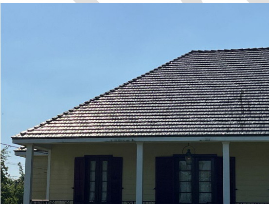
Figure 18: Example of synthetic slate roof
