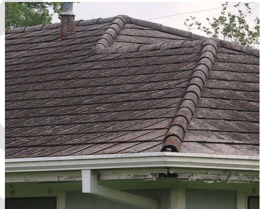
Figure 20: Example of an asbestos shingle roof
