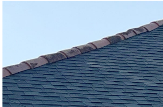
Figure 19: Example of a ridge tiles on an asphalt roof
