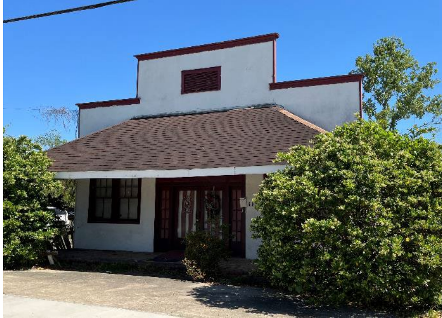
Figure 7- c.1930 Freestanding Commercial, 603 Main Street
