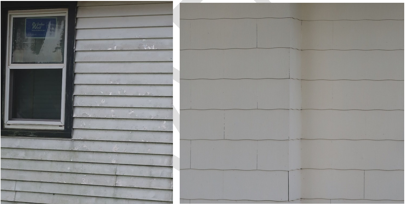
Figure 27: Example of aluminum siding (L) and asbestos shingle siding (R)
