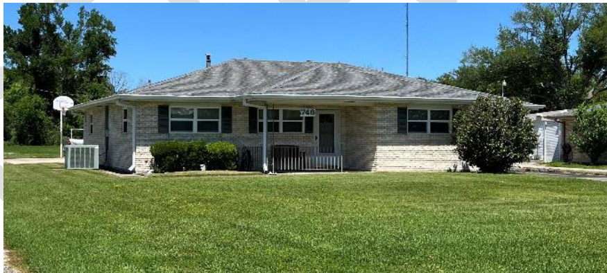
Figure 6- c.1965 Ranch, 748 West 5th Street
