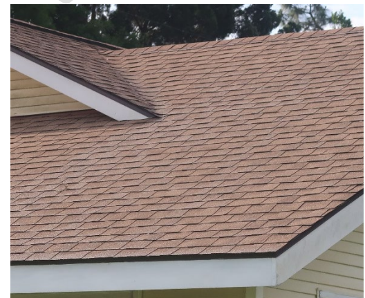
Figure 21: Example of an asphalt shingle roof.
