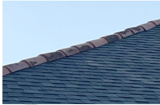
Figure 15: Example of a ridge tiles on an asphalt roof
