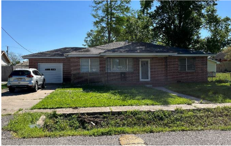
Figure 5- c.1960 Ranch, 120 North Church Street
