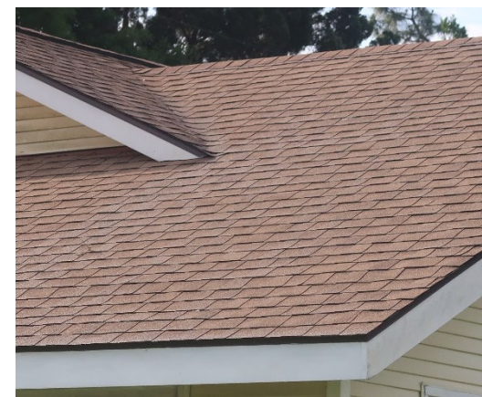
Figure 17: Example of an asphalt shingle roof.
