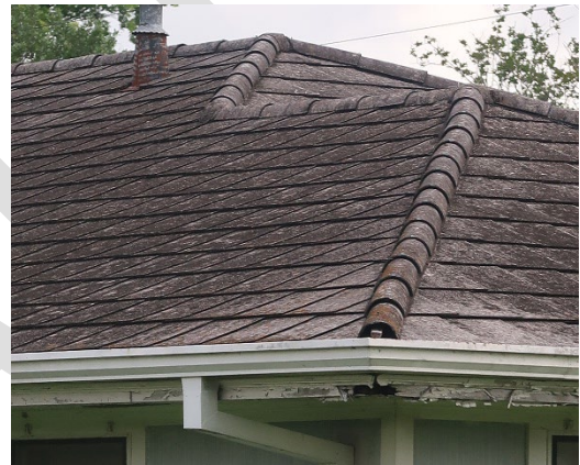
Figure 16: Example of an asbestos shingle roof
