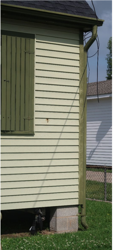
Figure 19: Example of a gutter and downspout
