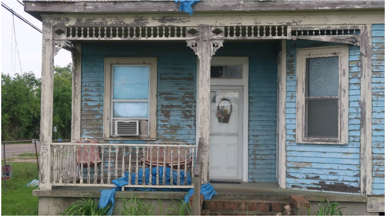
Figure 26: A porch with intact historic details.
