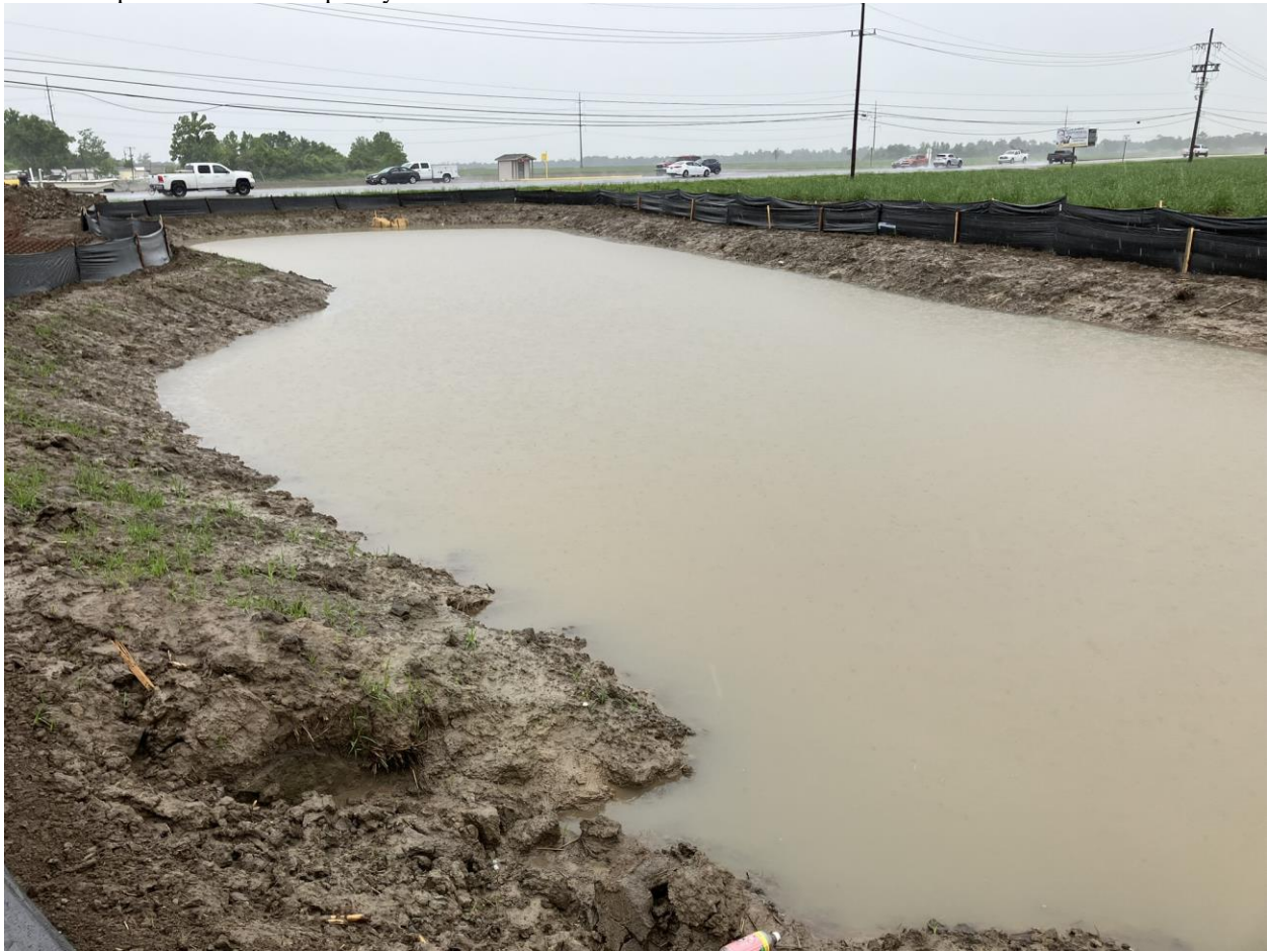
Detention pod – continue temporary stabilization
