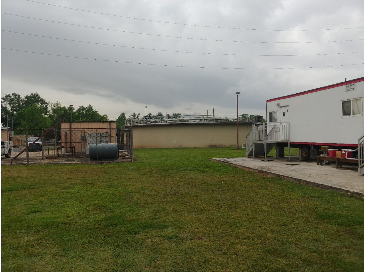
overall site looking south
