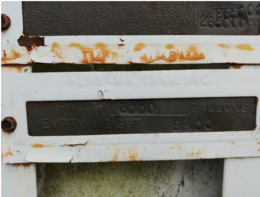
3,000 gallon diesel tank (double walled)
