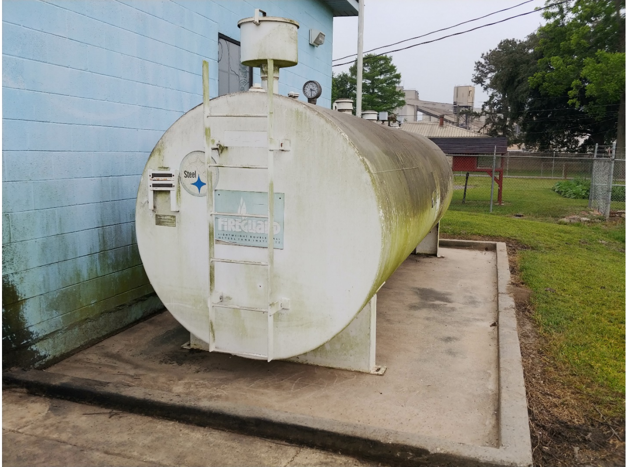
3,000 gallon diesel tank (double walled)
