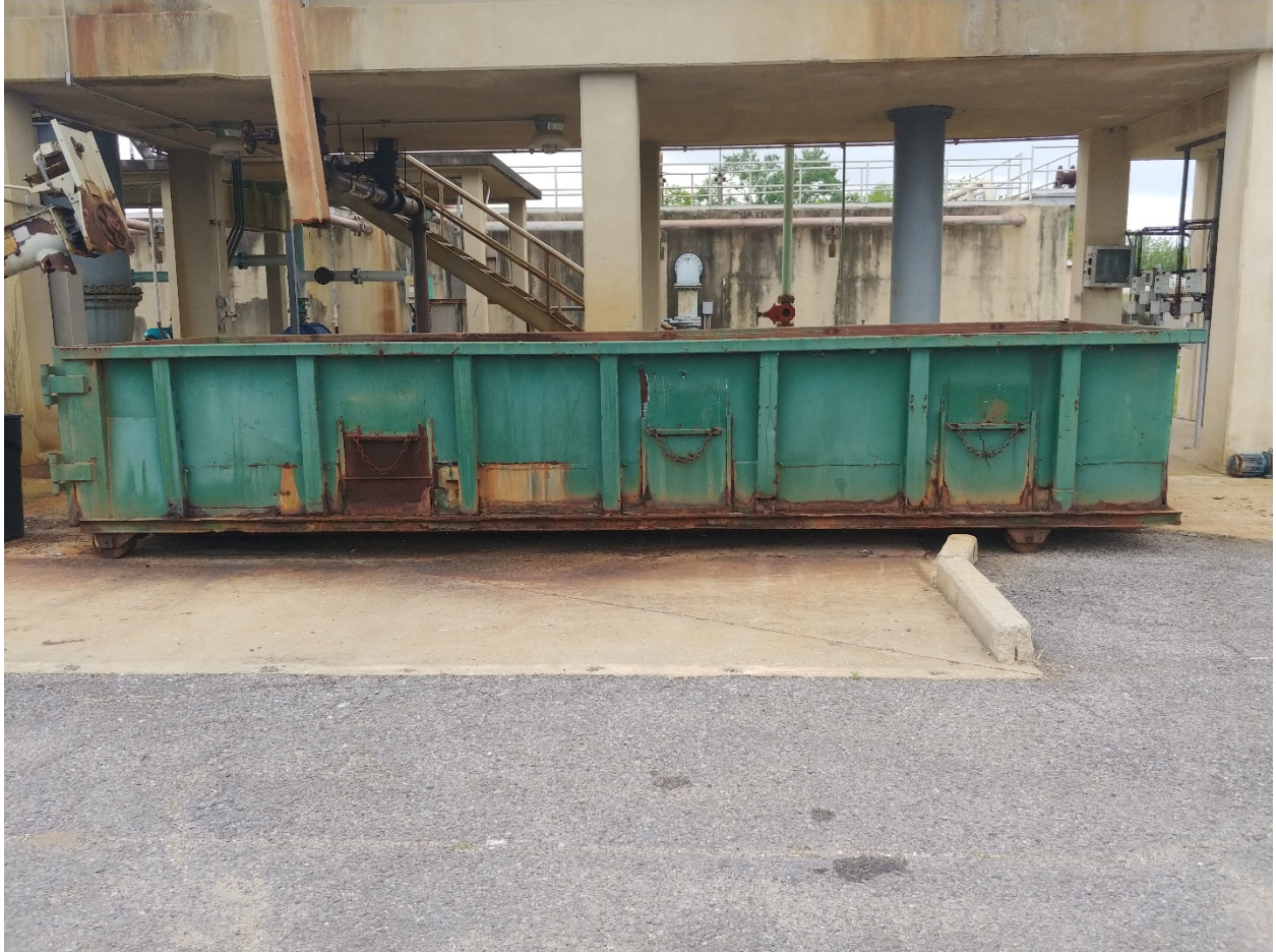
unused damaged rolloff box; drains to headworks
