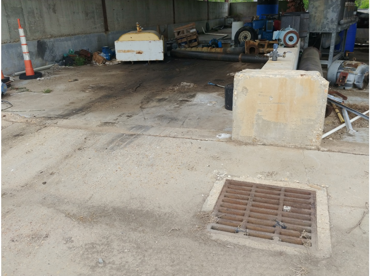
curb separates drying bed from nearest drain
